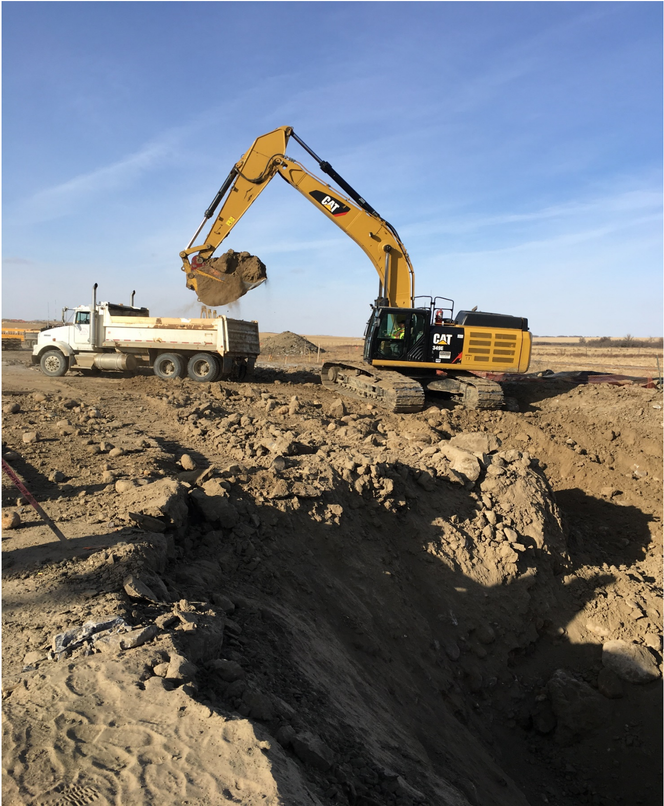
HAULING AWAY SOIL FROM ENTRY POINT
