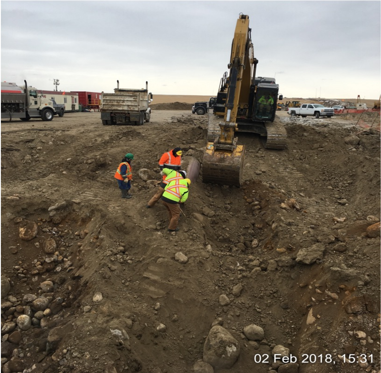
DIGGING OUT ENTRY POINT
