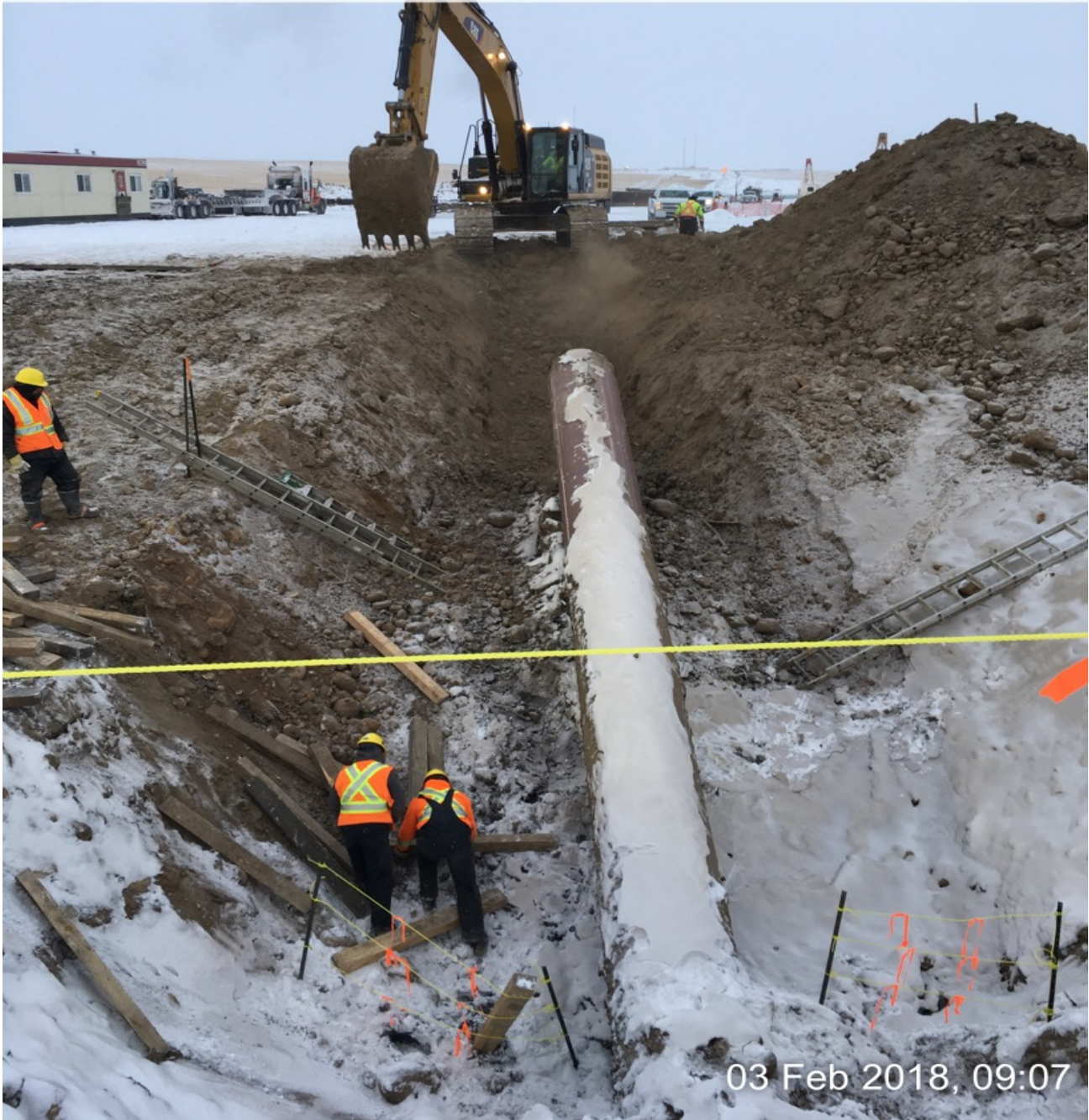
EXCAVATING PIPE AT ENTRY POINT
