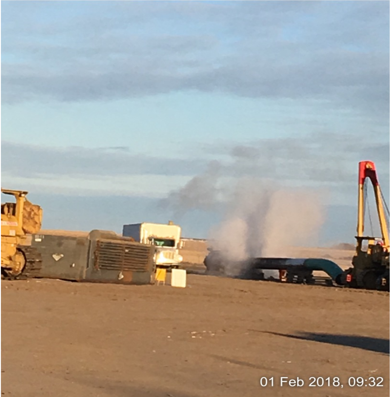
CLEANING PIPE SECTION
