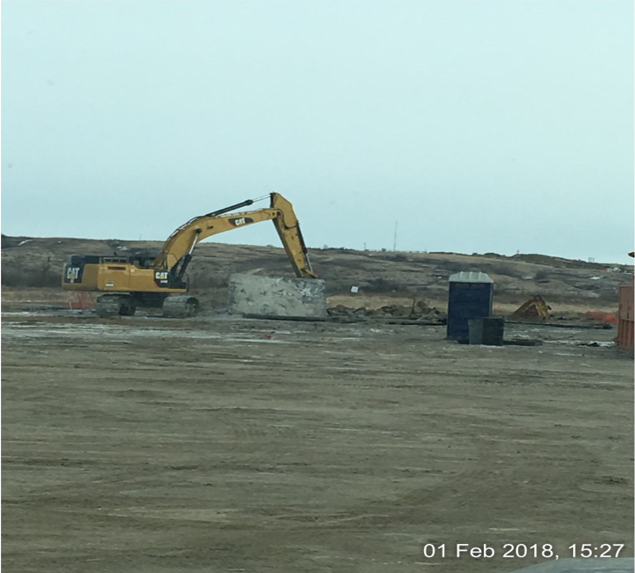
MOVING RIG MATS FROM RIG SITE
