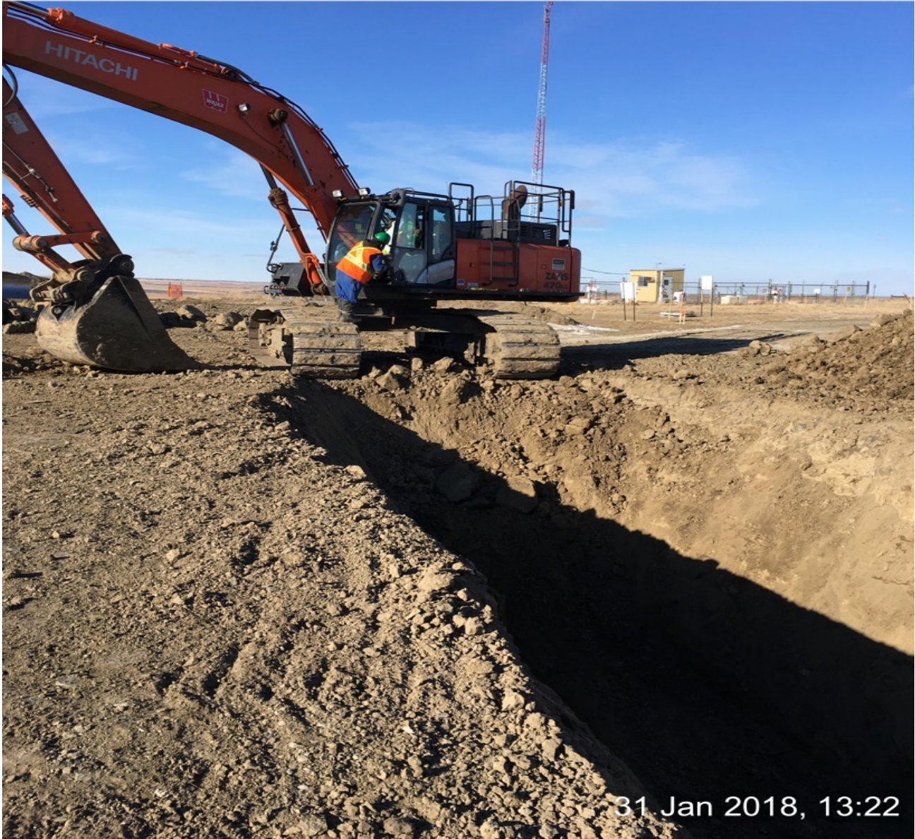
DIGGING DITCHLINE AT EXIT POINT
