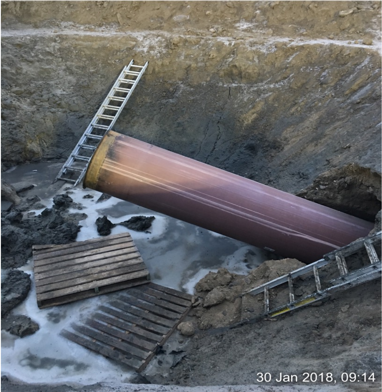
ENTRY POINT BEFORE EXCAVATION
