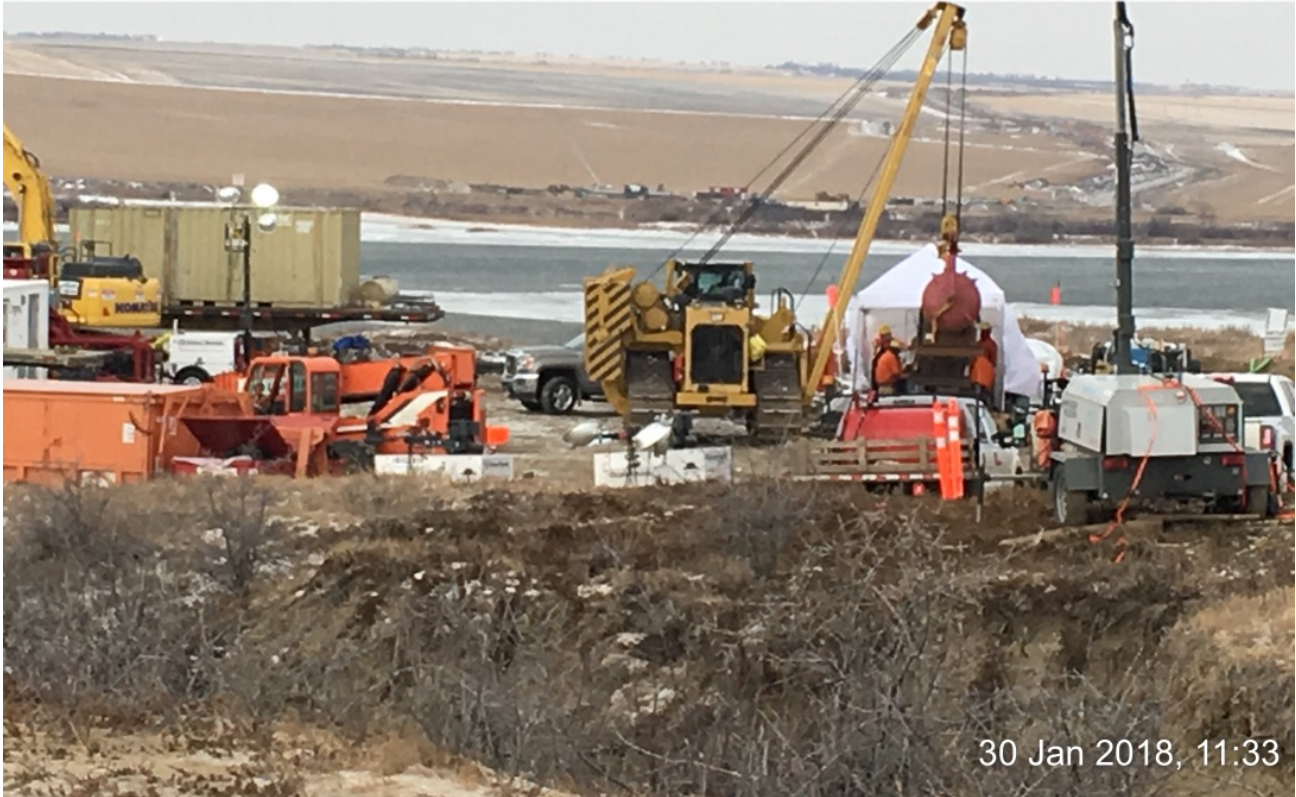
INSTALLATION OF TEST AT EXIT POINT
